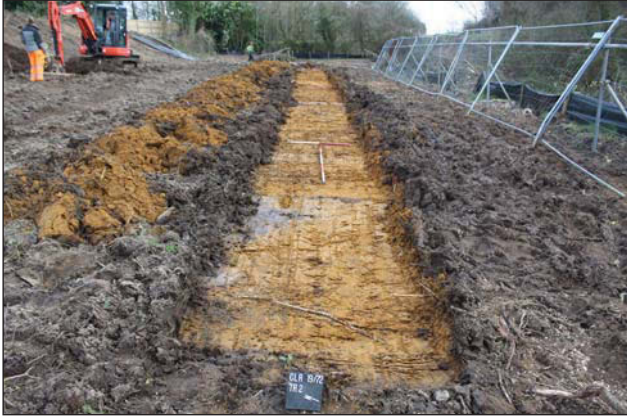
Plate 1. Trench 2, looking East, Scales: 2m, 1m and 0.2m.
