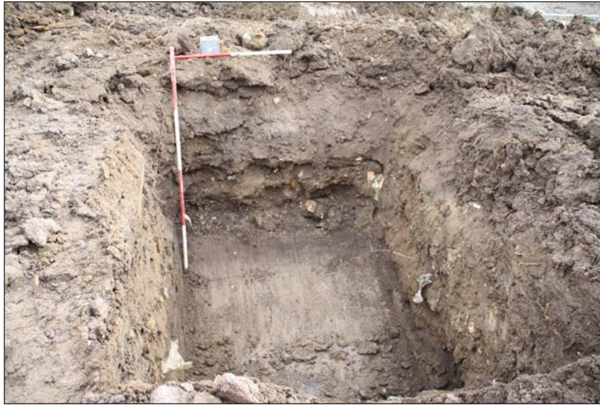
Plate 1. Manhole Trench 2, looking South East, Scales: 2m and 1m.
