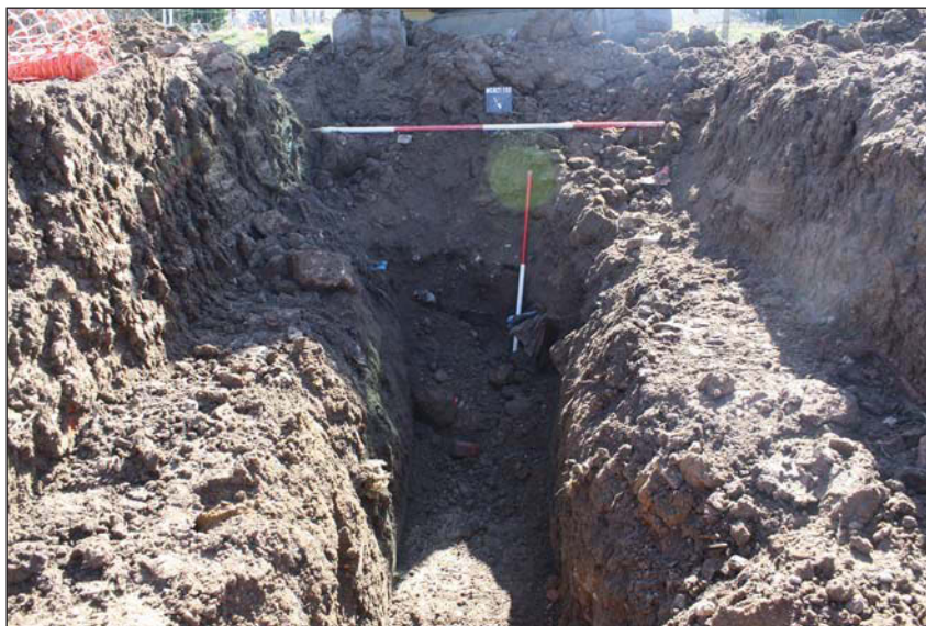
Plate 4. Main Pipe Trench, looking South East, Scales: 2m and 1m.
