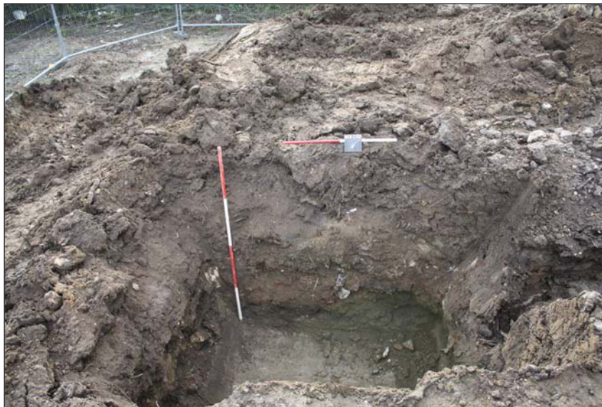
Plate 2. Pipe Trench, looking South East, Scales: 2m and 1m.
