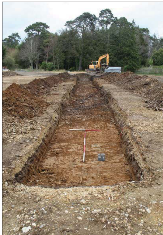
Plate 2. Trench 2, looking North, Scales: 2m, 1m and 0.3m.
