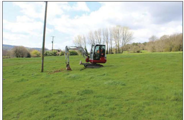
Plate 4. Trench 2, backfilled, looking West
