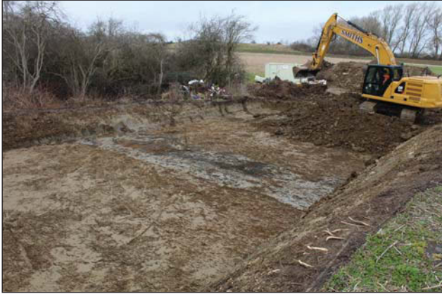
Plate 1. Access, modern ditch looking North West,
