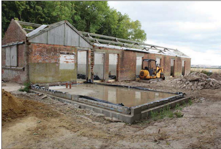
Plate 5. Barn 4, looking North East, new extension.
