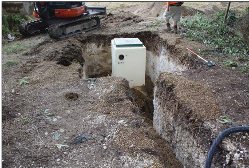
Plate 6. Barn 4, section of septic tank pit, looking South East, Scale: 1m
