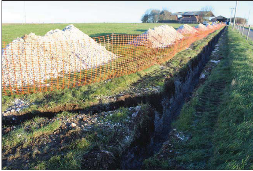
Plate 1. Service trench, looking north east towards Ilsley Barn Farm
