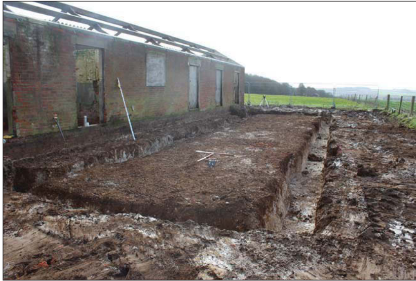
Plate 3. Barn 1, annexe footings, looking South East, Scales: 2m and 1m.
