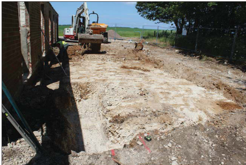
Plate 4. Barn 2, annexe reduction and footing, looking North West.
