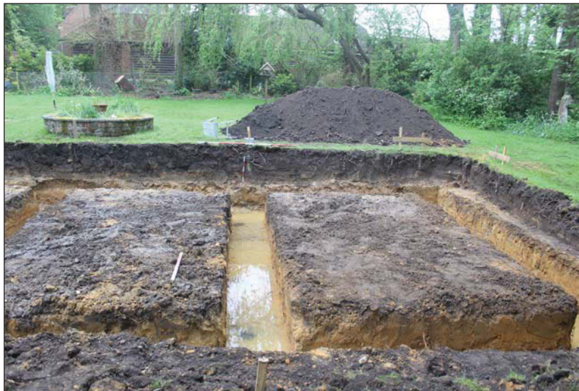
Plate 2. Section view, looking south-east, Scales: 2m, 1m and 0.5m.
