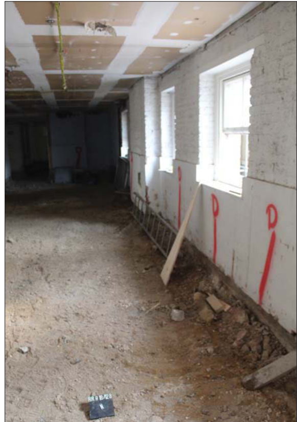
Plate 2. Ground reduction- interior, south end, looking north
