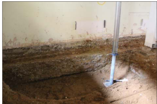
Plate 3. Test Pit 1. looking north
