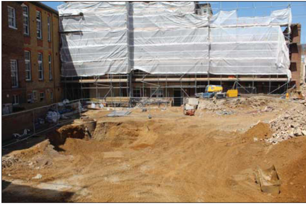
Plate 1. Ground reduction- exterior looking west
