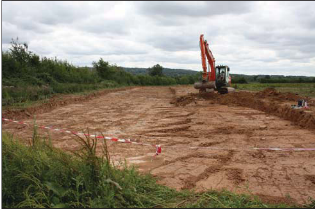
Plate 1. Site during initial strip, looking south.
