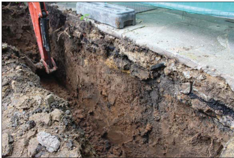
Plate 2. New foundation trench during excavation looking south west.
