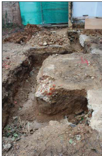
Plate 3. Former foundation trench after removal of footings, looking west
