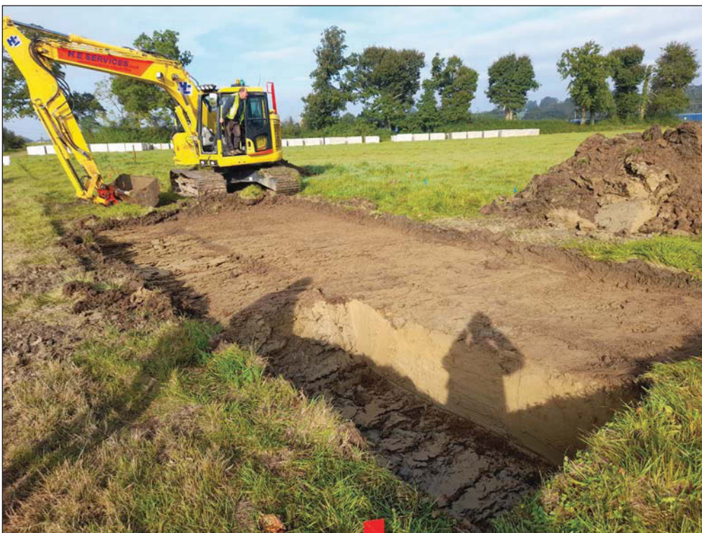
Plate 2. Ground reduction for substation 2 and warehouse, looking north, with test pit.
