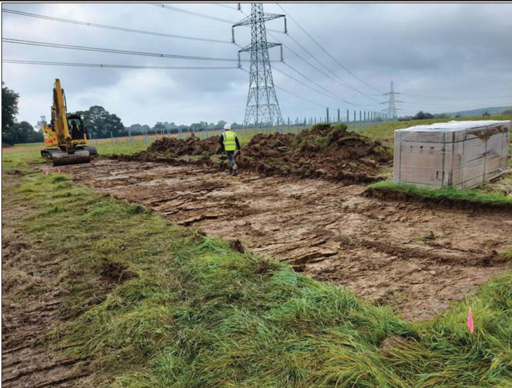
Plate 1. Ground reduction for substation 1 and warehouse, looking south.
