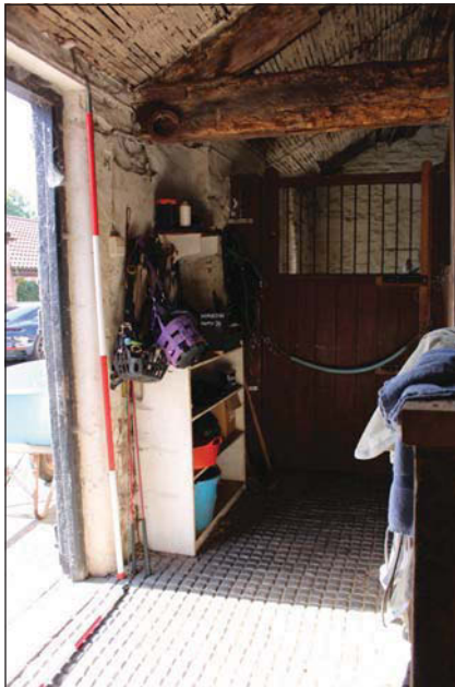
Plate 17. South wall, looking West. Scales: 1x1m and 1x2m.
