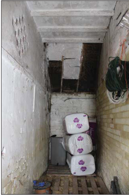
Plate 5. General photo to north wall, looking North.
