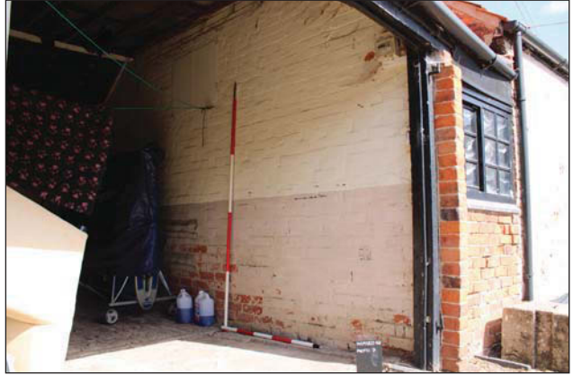
Plate 14. Building 1A, west wall, looking North East. Scales: 1x1m and 1x2m.
