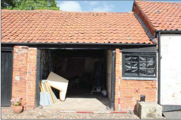
Plate 13. Building 1A, front elevation, looking North. Scales: 1x1m and 1x2m.
