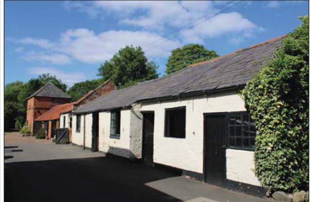
Plate 2. Stable block and dovecote, looking North West.
