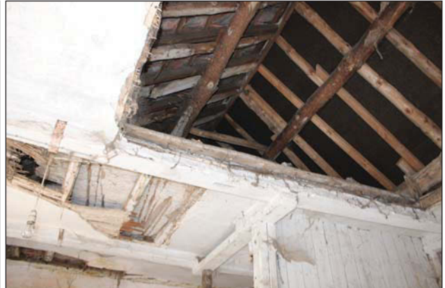
Plate 12. Roof construction, looking West.
