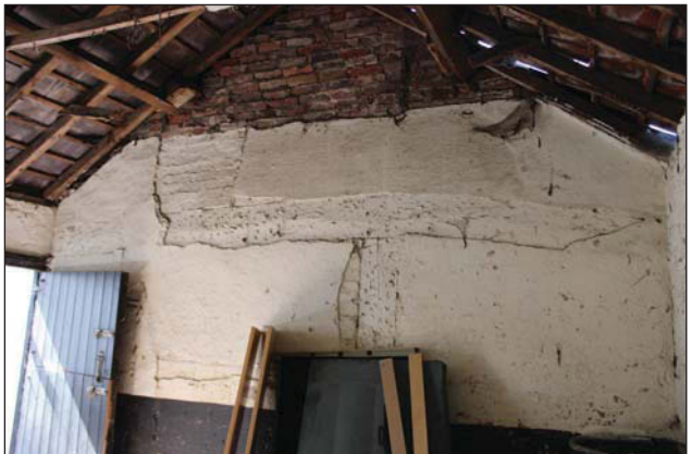
Plate 28. West wall showing timbers, looking West.
