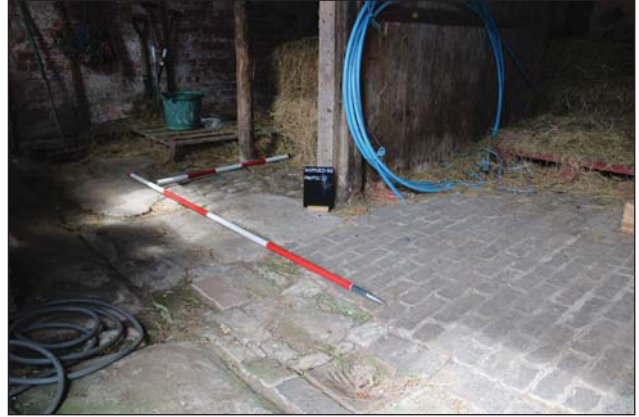
Plate 10. Floor detail, looking North West. Scales: 1x1m and 1x2m.
