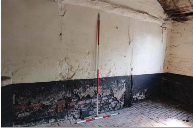
Plate 21. East wall showing timbers, looking South East. Scales: 1x1m and 1x2m.
