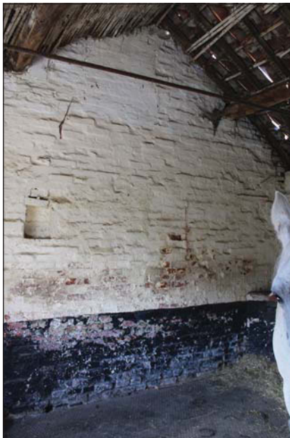
Plate 19. West wall, looking North West.
