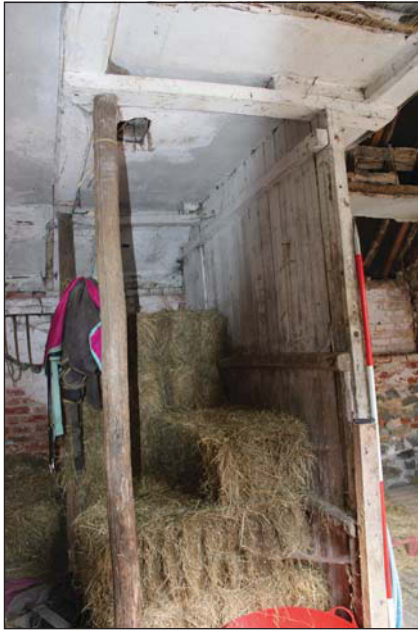
Plate 9. Stud wall and post, looking North East. Scale: 1x2m.
