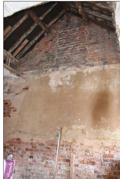
Plate 8. East gable end wall showing blocked pitching eye. Looking North East.
