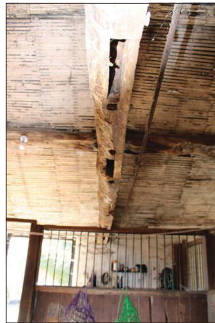
Plate 24. View along beam showing reuse, looking South.
