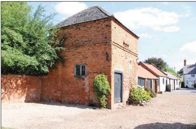
Plate 3. Dovecote, looking North East.
