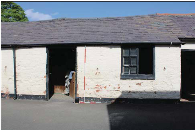
Plate 15. Building 2, front elevation, east end, looking North. Scales: 1x1m and 1x2m.
