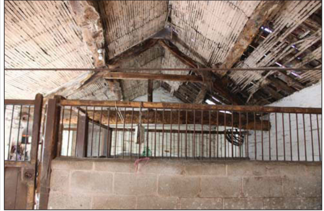
Plate 22. Roof construction, looking West.
