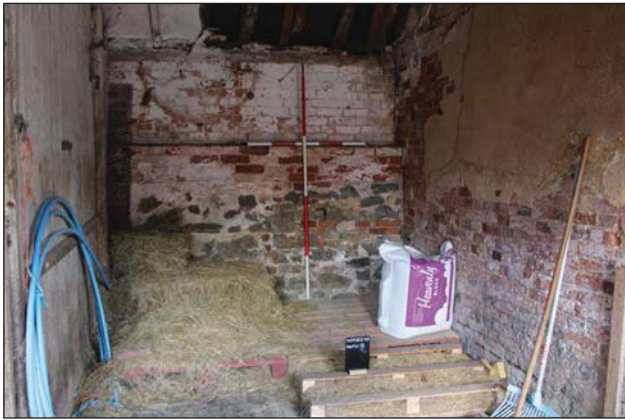
Plate 7. North wall, east end, looking North. Scales: 1x1m and 1x2m.
