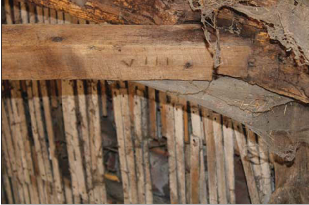
Plate 25. Carpenters mark detail 'VIII', looking West.
