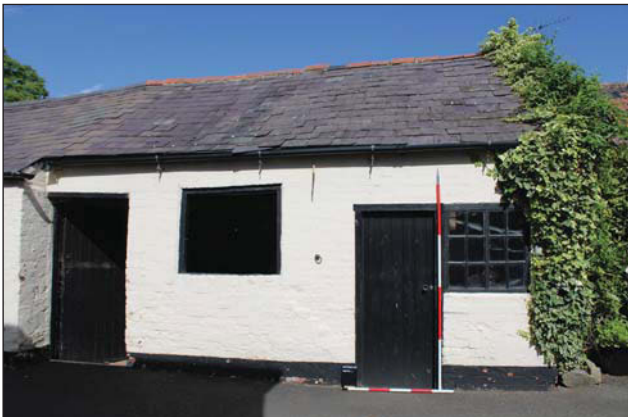
Plate 27. Building 3, front elevation, looking North. Scales: 1x1m and 1x2m.
