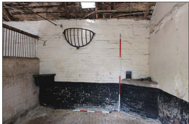
Plate 20. North wall, east end, looking North. Scales: 1x1m and 1x2m.
