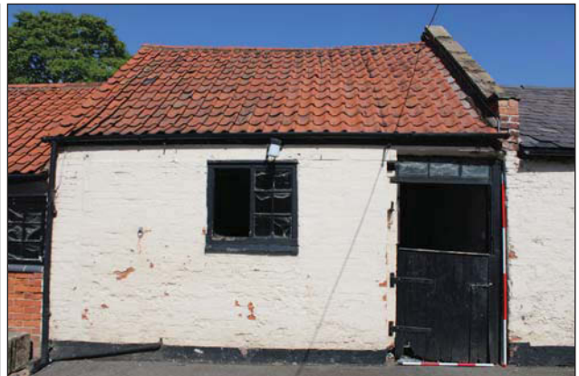
Plate 4. Building 1, front elevation, looking North, Scales: 1x1m and 1x2m.
