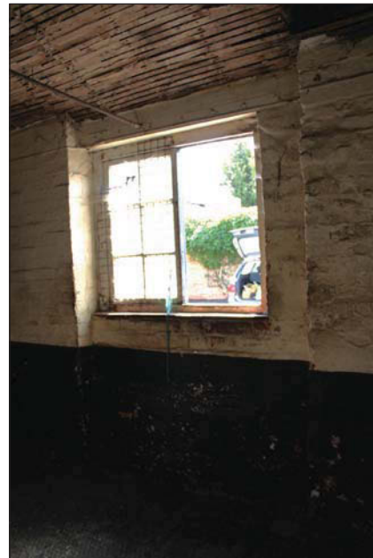
Plate 18. South wall, west end, window, looking West.
