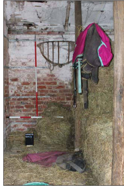
Plate 6. North wall, west end, looking North. Scales: 1x1m and 1x2m.
