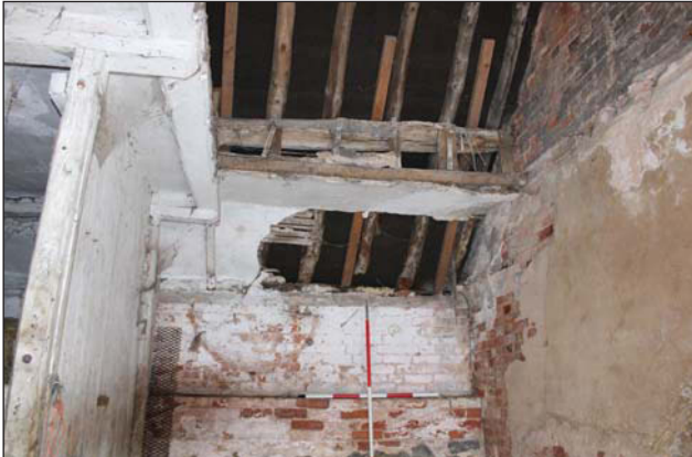
Plate 11. Roof construction, looking North. Scales: 1x1m and 1x2m.
