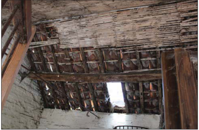
Plate 26. Roof detail, looking North.
