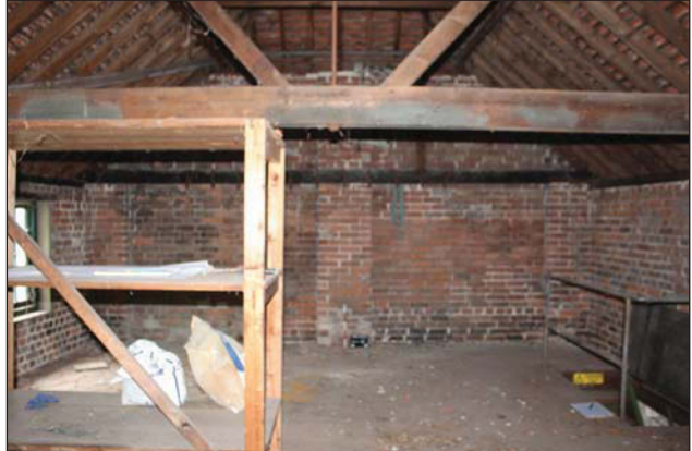
Plate 18. South gable end looking South; Scale:0.5m.
