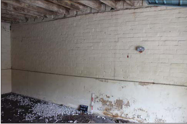
Plate 9. Garage, Oblique view to south wall looking South East; Scale: 0.5m.
