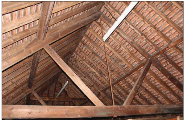
Plate 20. Roof detail, looking North East.
