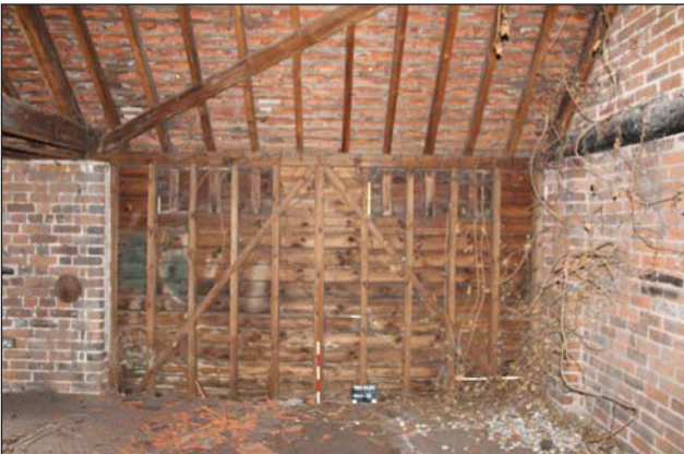
Plate 15. Room 5, Weatherboarding, internal view, looking West; Scale: 0.5m.
