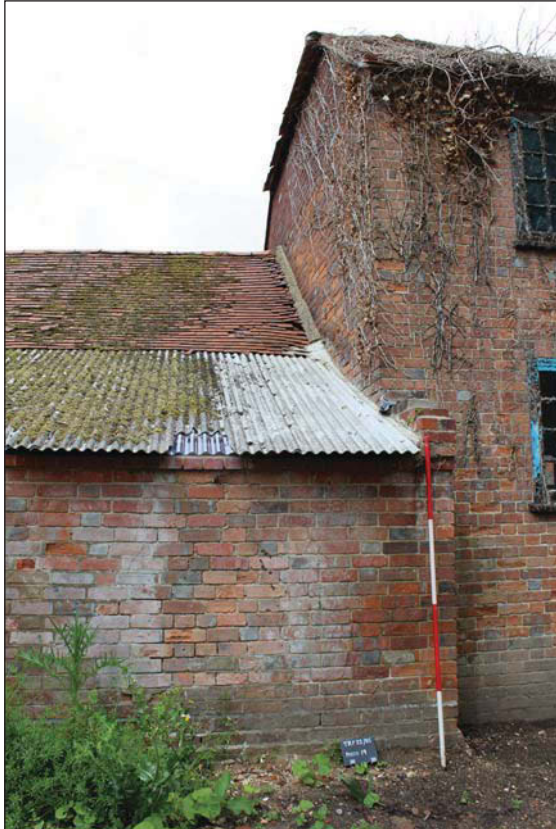
Plate 25. Rear, centre, looking West; Scale: 2m.
