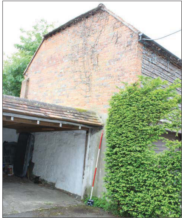
Plate 6. Oblique to northern gable end, looking South East.
