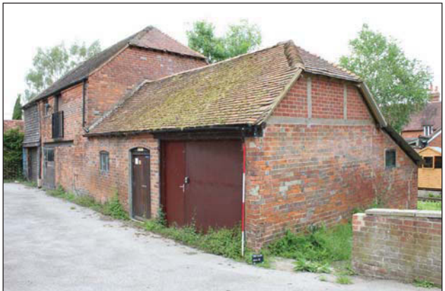
Plate 4. Southern gable end, oblique, looking North East; Scale: 2m.
