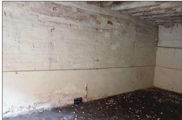
Plate 8. Garage, Oblique view to north wall, looking North East; Scale: 0.5m.
