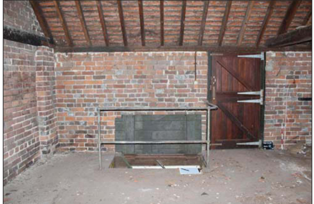
Plate 14. Room 5, Stair opening, looking West; Scale: 0.5m.
