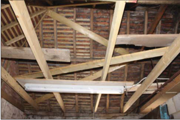
Plate 33. Room 4, Roof detail, looking West.
