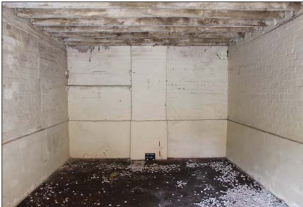
Plate 7. Garage, East wall, looking East; Scale:0.5m.
