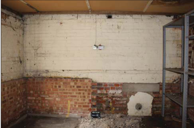
Plate 29. Room 3, North wall, looking North, Scale: 0.5m.
