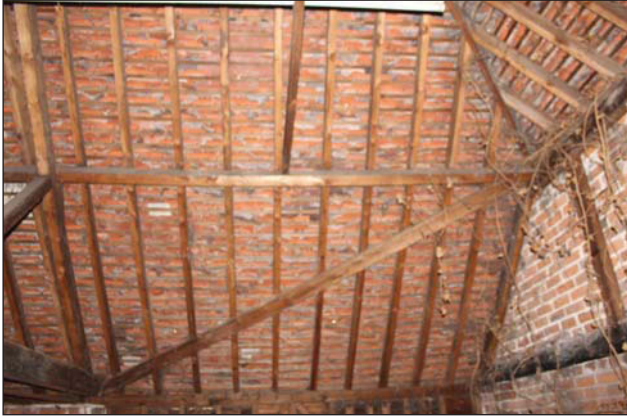
Plate 21. Roof detail, room 5, looking West.
