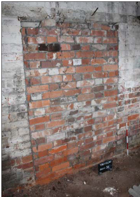
Plate 27. Room 2 Blocked door to room 3, looking West; Scale: 0.5m.
