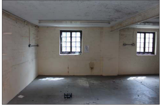
Plate 10. Room 1, View to window looking East; Scale: 0.5m.
