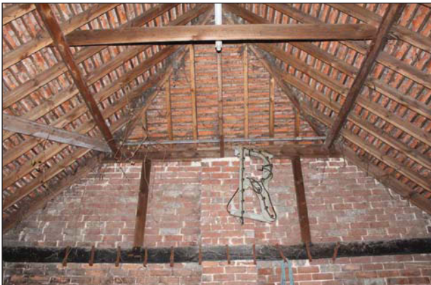
Plate 19. Hip detail, looking South.
