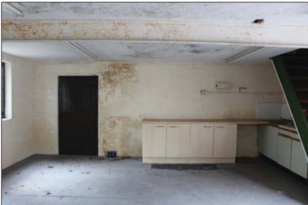
Plate 11. Room 1, View to door to room 2 looking South; Scale: 0.5m.
