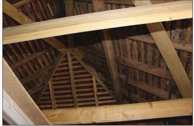
Plate 34. Room 4, Hip detail, looking South.
