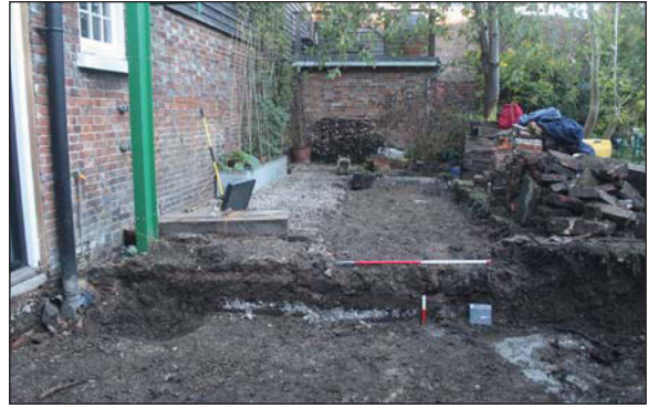
Plate 2. General view of site during initial ground reduction, looking East. Scales: 1m and 0.20m.
