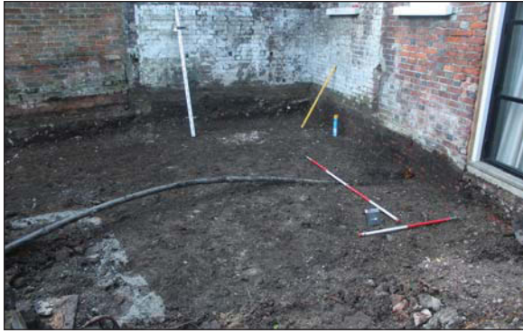
Plate 1. General view of site during initial ground reduction, looking North-west. Scales: 2m and 1m.
