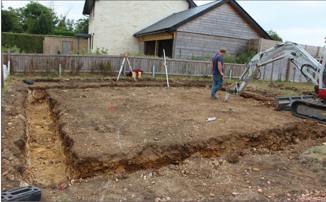
Plate 1. Garage foundation trenches, general view, looking north west.
