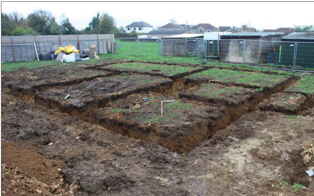
Plate 2. House foundation trenches, looking east, Scales: 2m and 1m.
