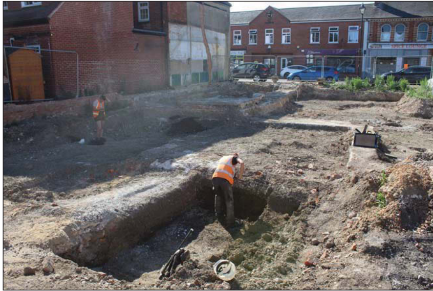
Plate 3. Excavation area, looking South.
