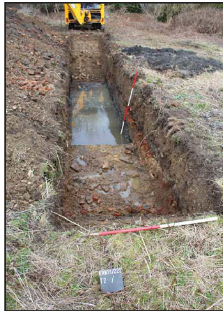
Plate 2. Trench 2, looking north west, Scales; 2m and 1m
