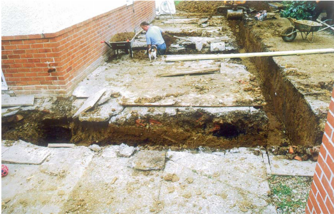
Plate 1. General view over footings, looking north east.
