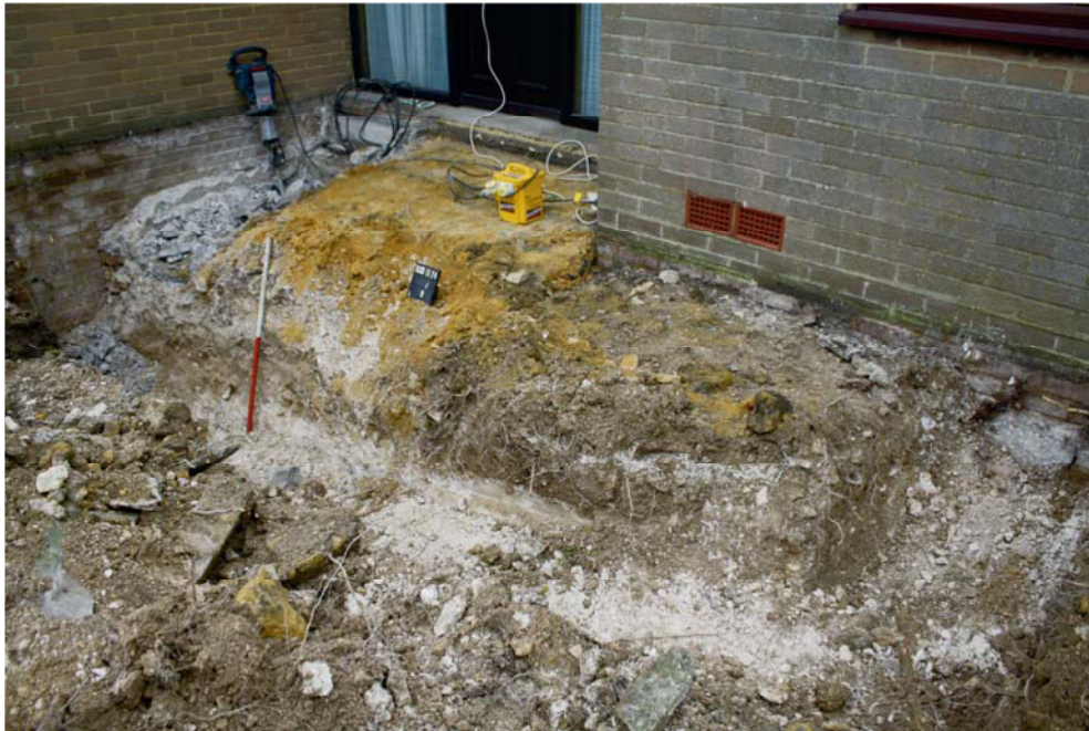
Plate 1. North footing trench, looking south-east, Scale: 1m
