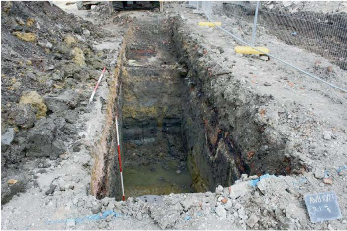
Plate 1. Trench 1, looking north east, Scales: 2m
