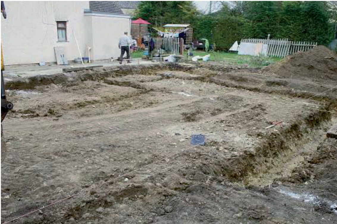
Plate 1. General shot looking north east over footing trenches.
