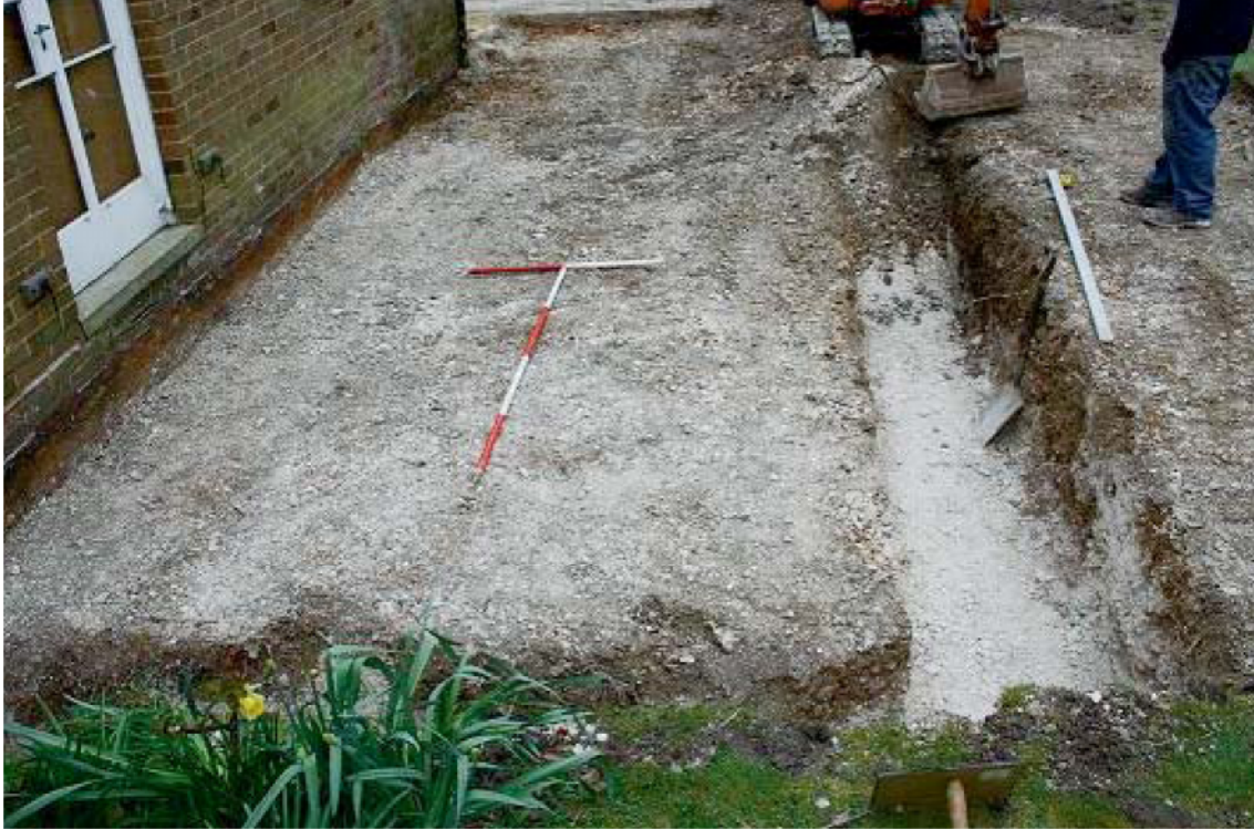
Plate 1. Ground reduction and trench footing, looking north, Scales: 2m and 1m.
