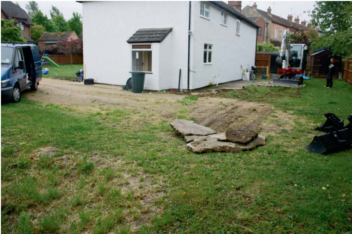
Plate 1. Area of rear and east extension, before footing excavation.
