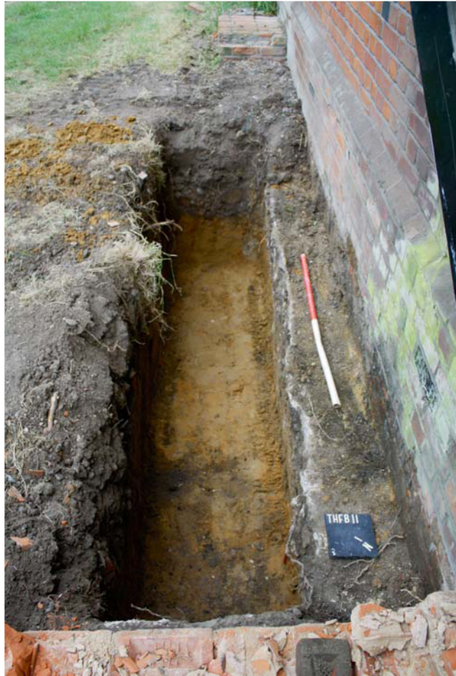
Plate 1. Footing trench looking south-west. Scale: 1m.
