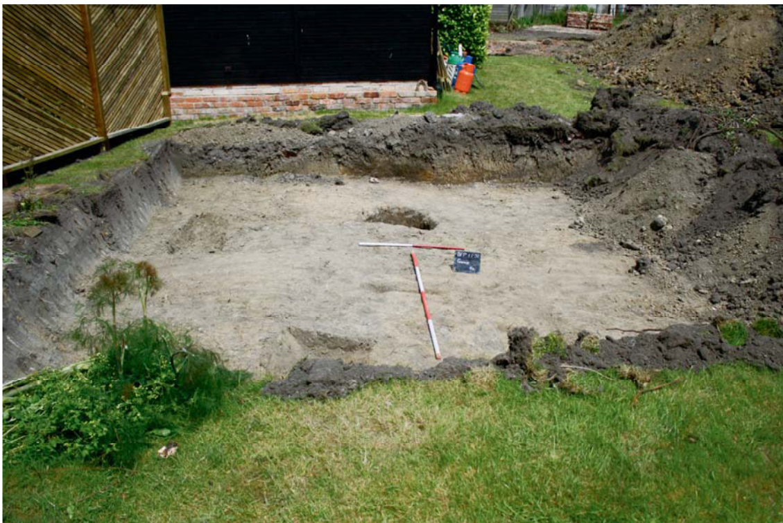
Plate 3. Area of Garage excavation, looking north east, scales 2m and 1m.
