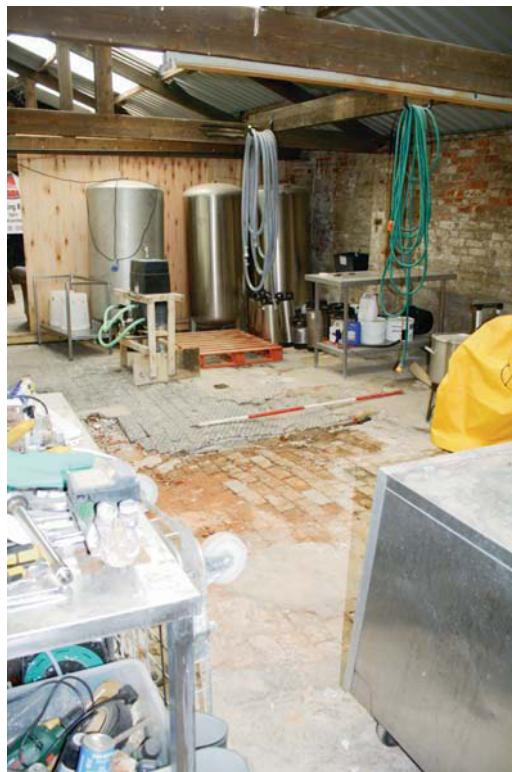
Plate 4. General view of room in NW corner of extension, looking SW; Scale: 2m
