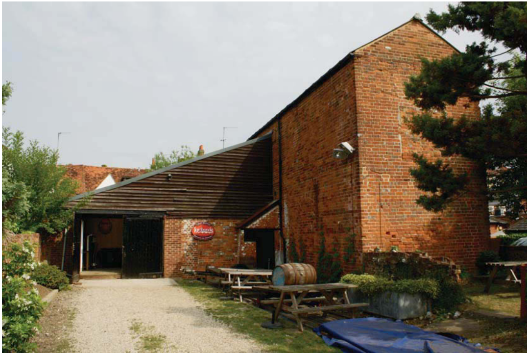
Plate 1. Exterior, general view, looking north
