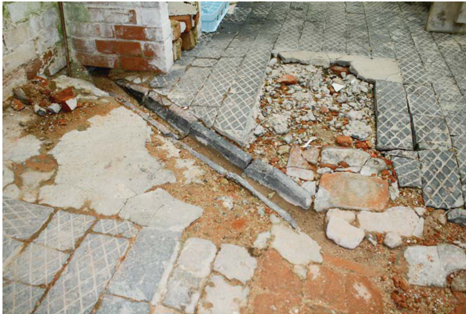
Plate 3. Detail of drain, looking east
