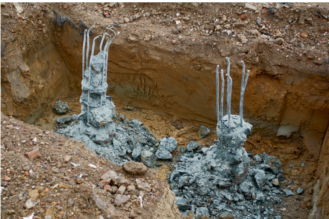
Plate 2. Pile cap in the centre of the site.
