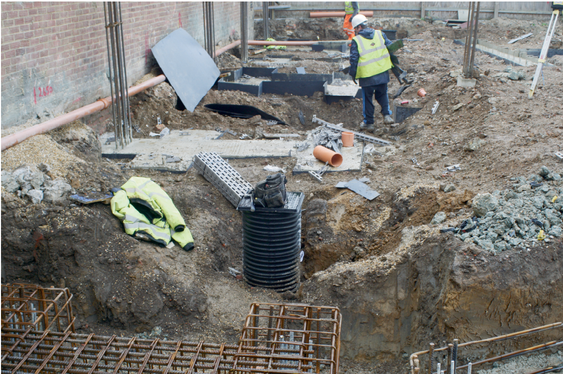
Plate 1. Pile caps on the eastern edge of the site.
