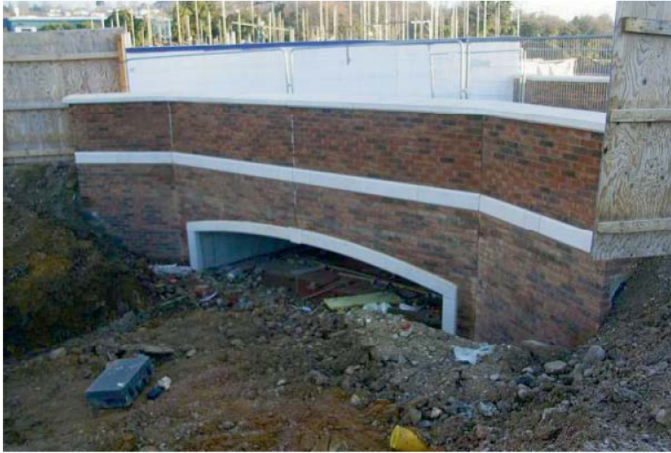
Plate 4. Constructed bridge looking east, with culvert level in foreground.
