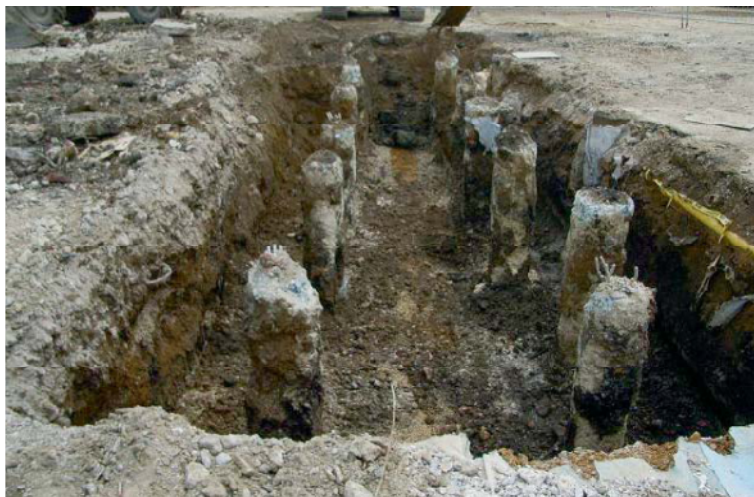
Plate 3. Bridge support area looking east.
