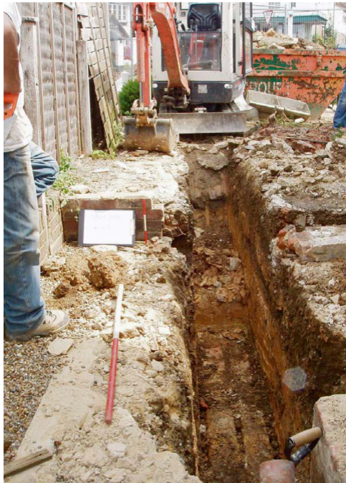
Plate 2. New footing trench, looking east. Scales: 1m and 0.3m
