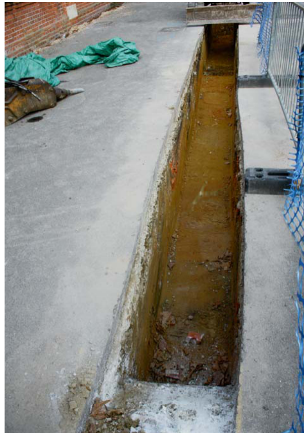
Plate 2. Footing trench, looking north east.
