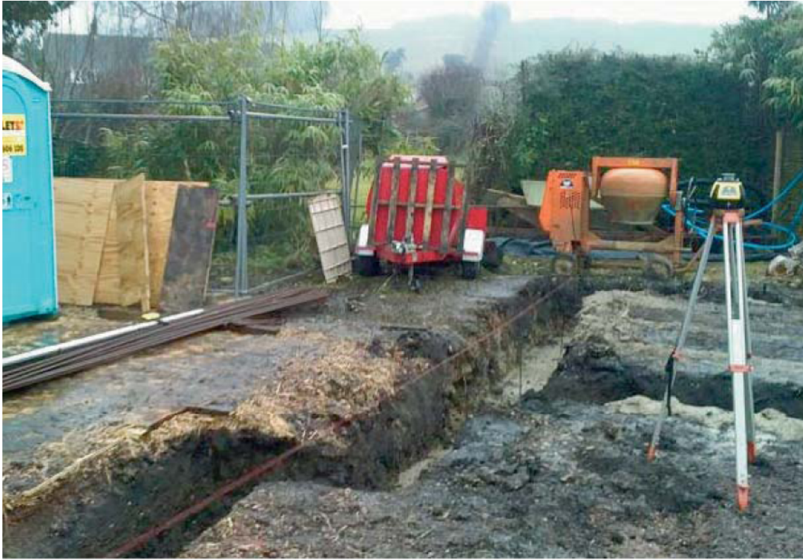
Plate 1. General site shot, looking east.
