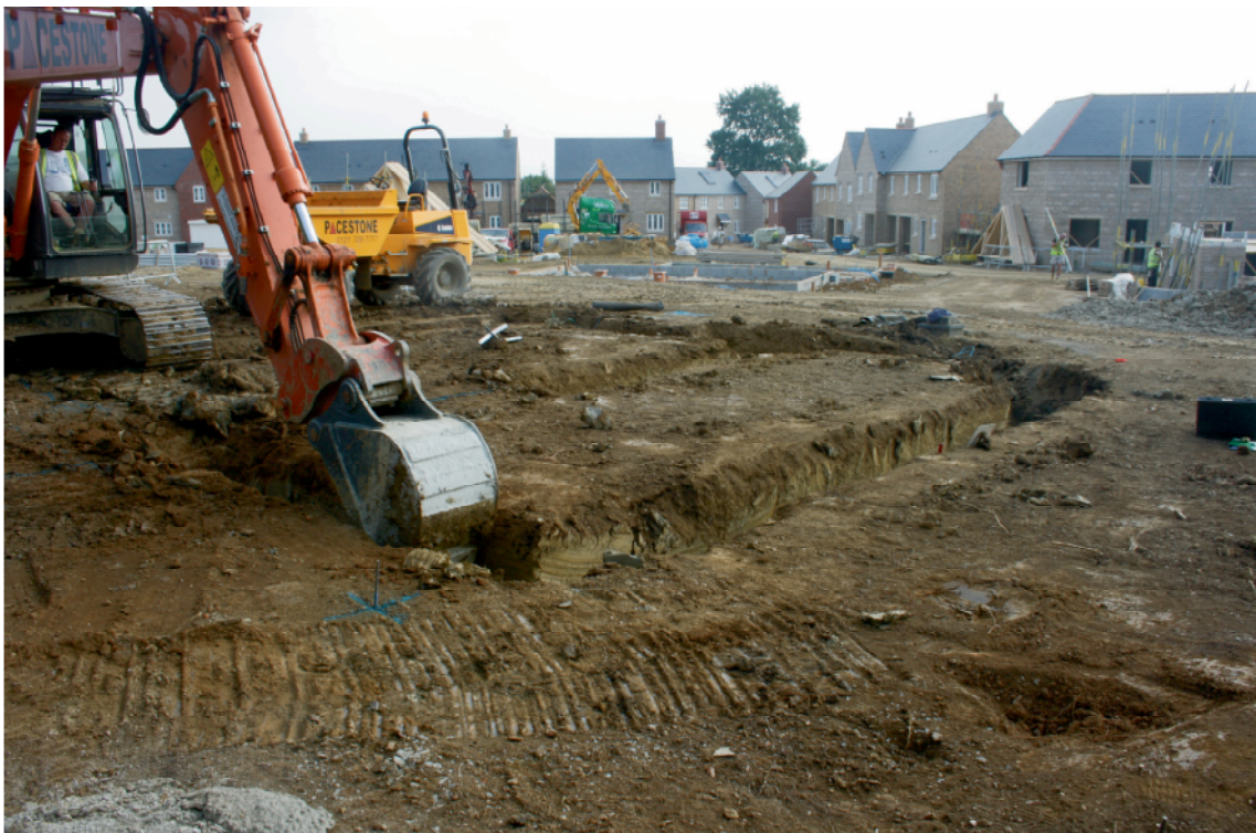
Plate 2. Plot 33 under excavation.
