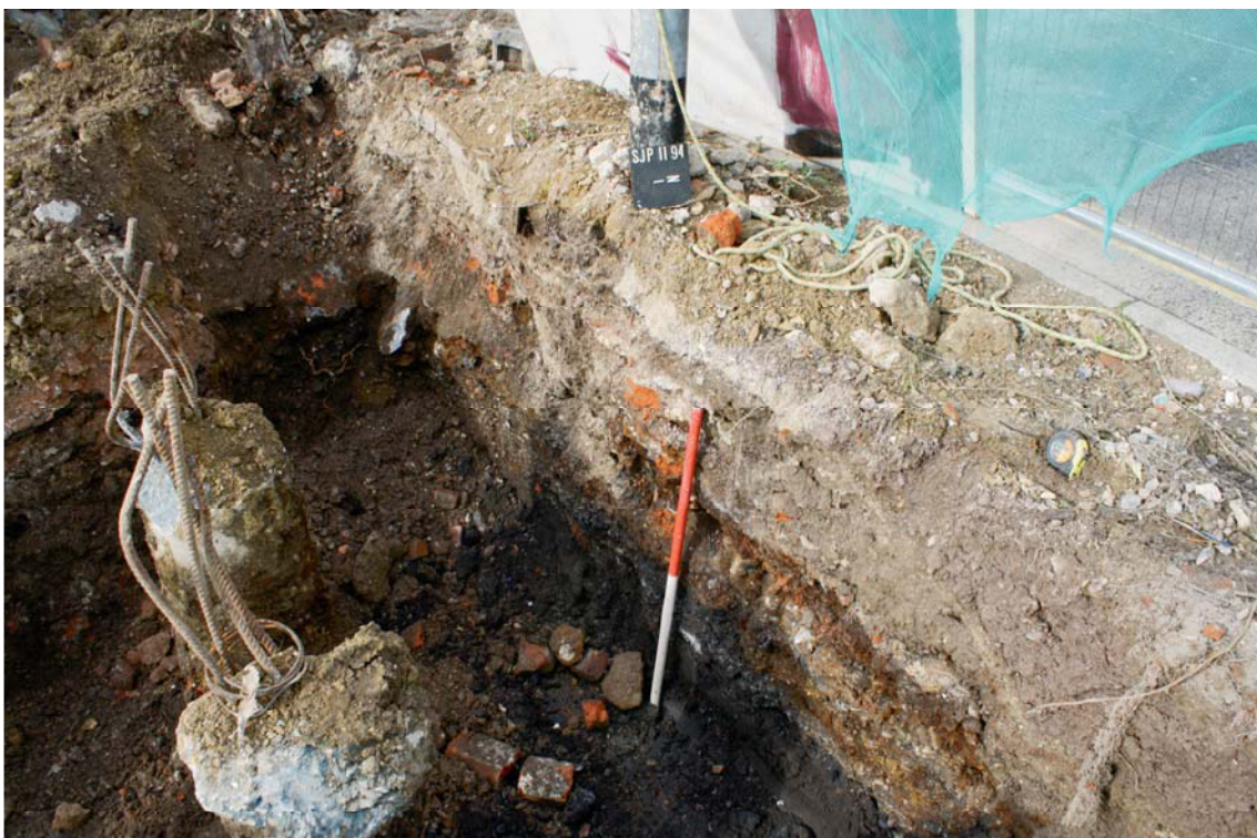
Plate 2. NE corner of dug footing, looking north, Scale: 1m.
