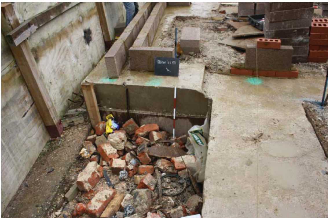
Plate 2. Imported modern rubble with new foundation, looking east.
