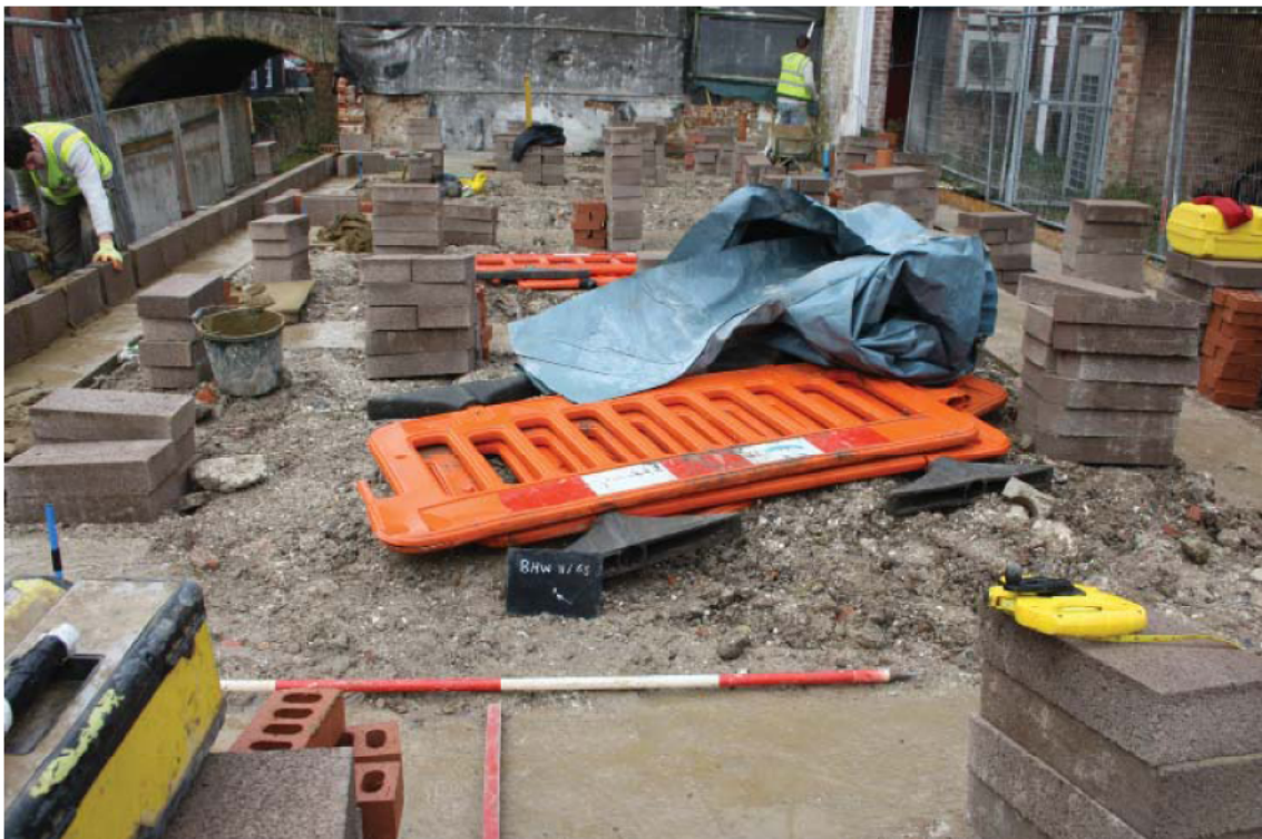
Plate 1. General site condition, looking east
