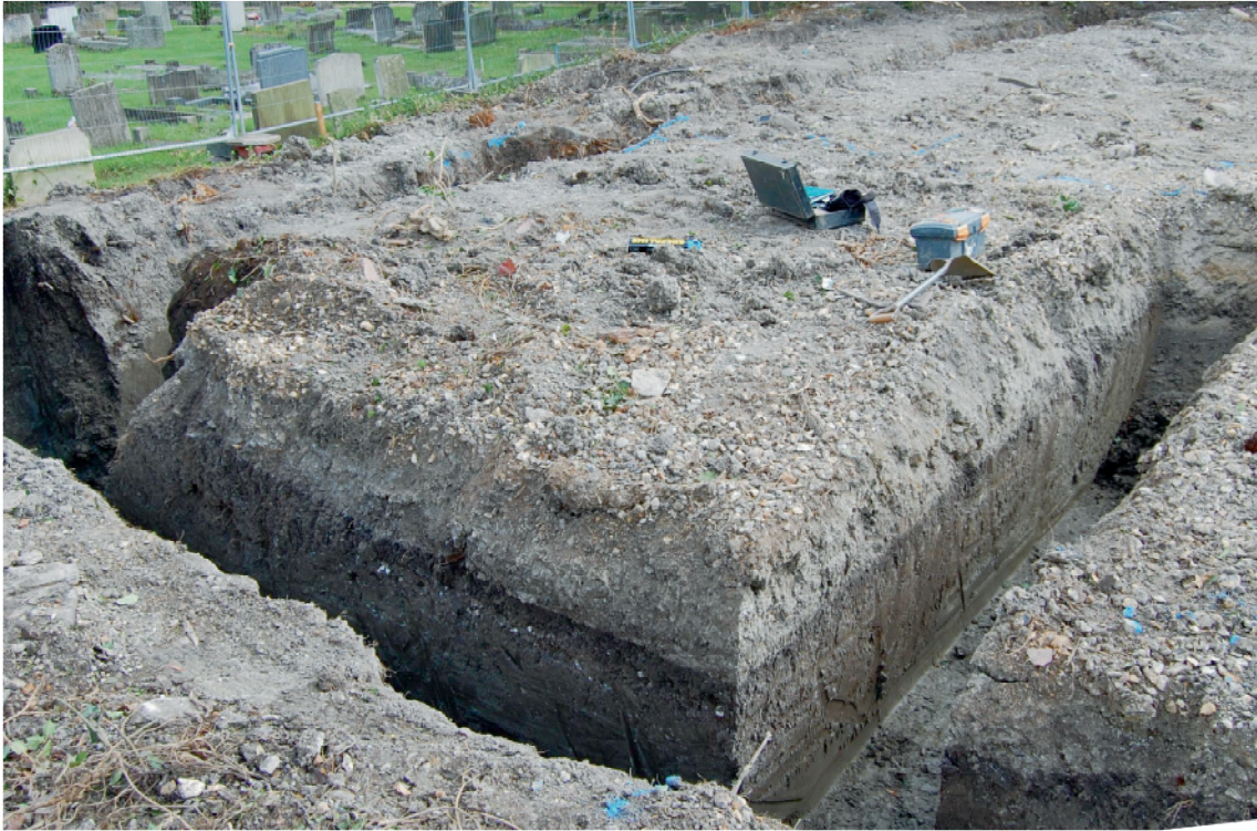
Plate 1. General shot over new footings.
