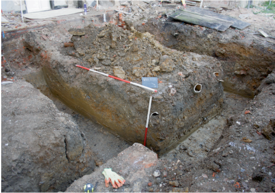
Plate 1. The excavated footings, looking south west, Scales: 2m and 1m.
