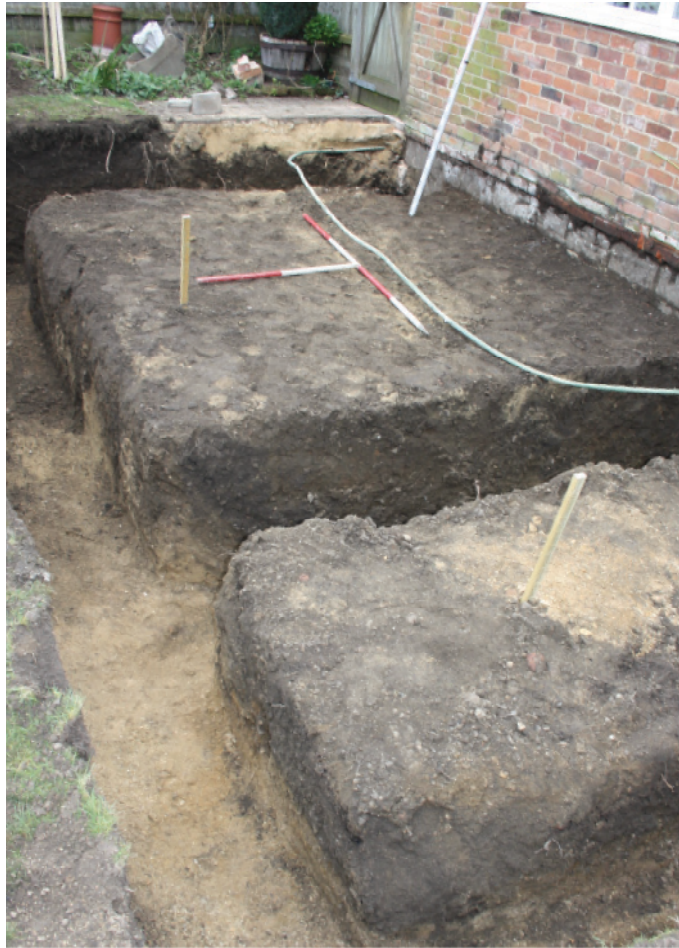
Plate 1. New footings, looking north east Scales: 2m and 1m.
