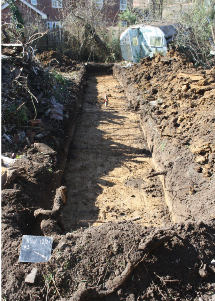
Plate 3. Trench 3 looking west. Scale: 2m
