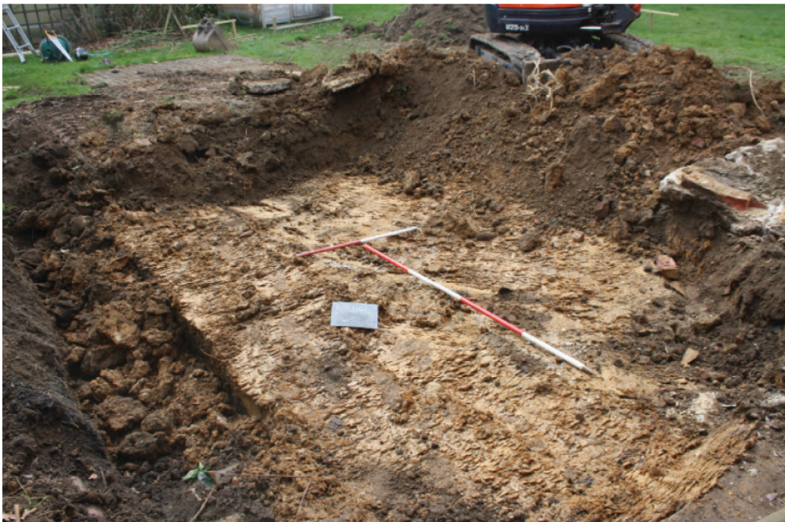
Plate 1. Reduced level for swimming pool to top of natural geology, looking south, Scales: 2m and 1m.
