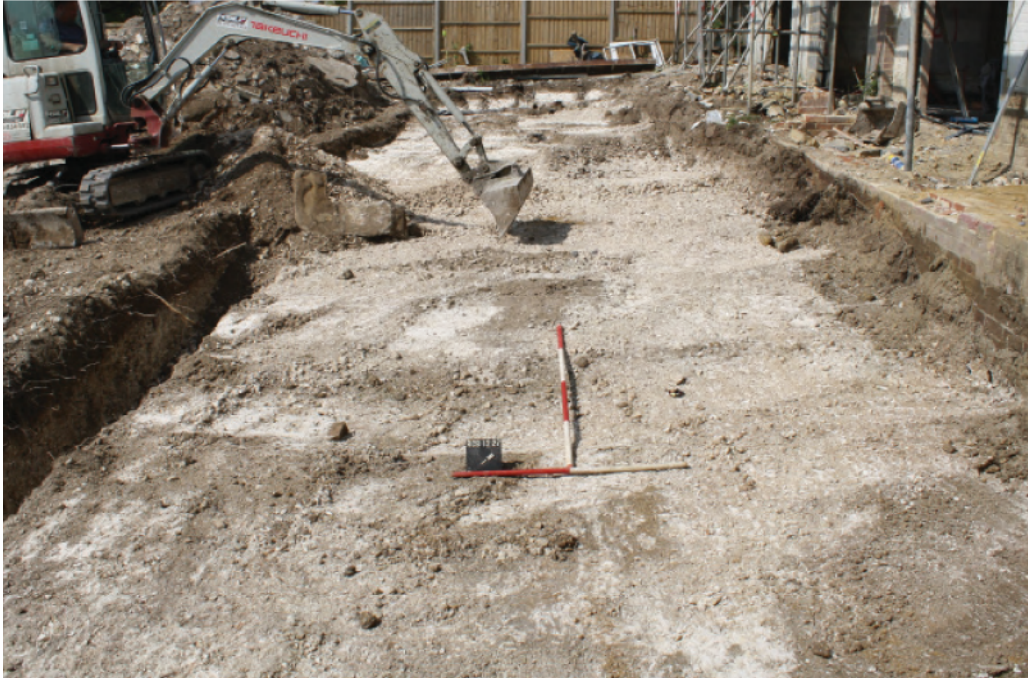
Plate 1. General site shot, looking north west: Scales: 2m and 1m.
