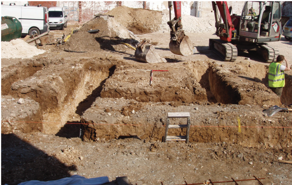
Plate 1. Block A under excavation, looking south, Scale:s 2m and 1m.
