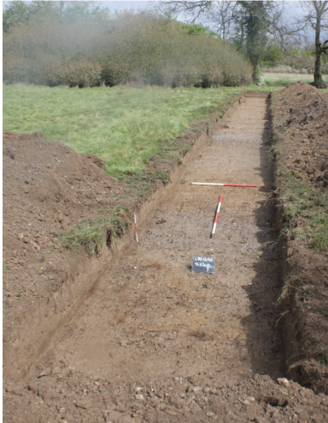
Plate 1. Trench 33, looking north, Scales: 2m and 1m.
