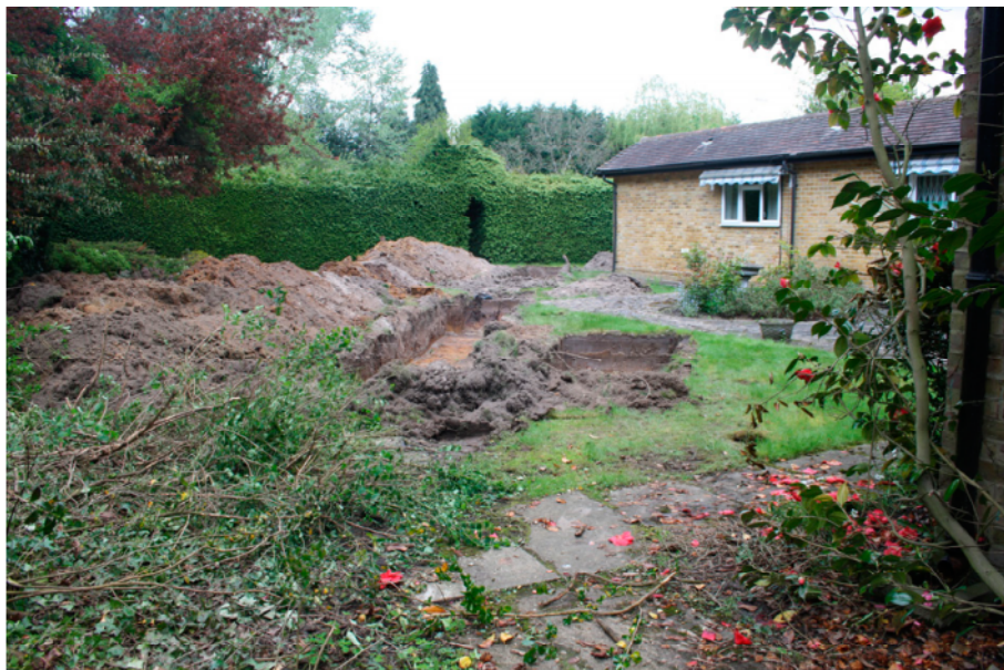
Plate 2. General view of the site, looking north.
