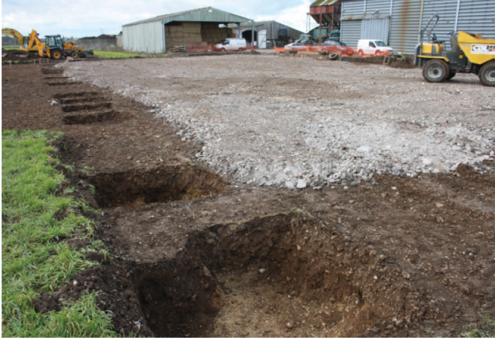
Plate 1. Pad excavation, looking north-west, from south-eastern corner pad.
