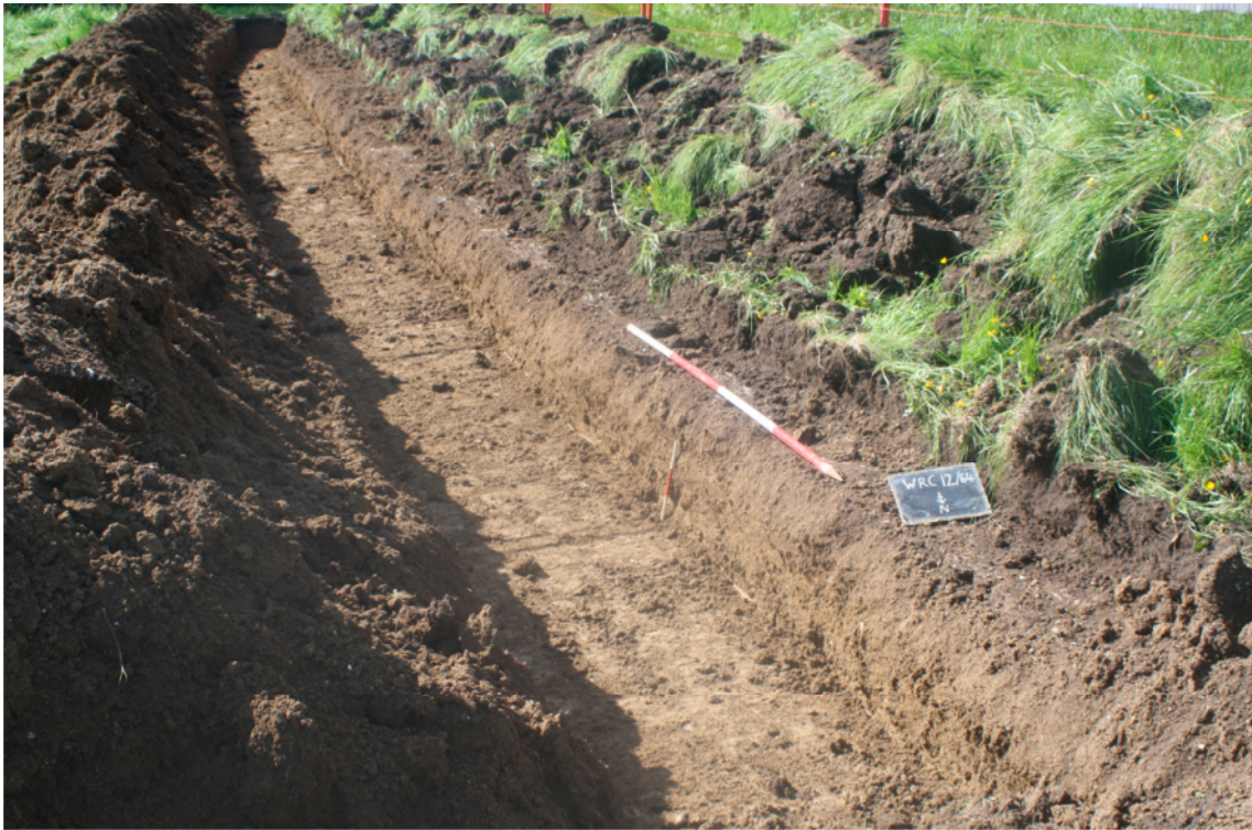
Plate 1. Pipe trench, looking southwest, Scales: 2m and 0.3m.
