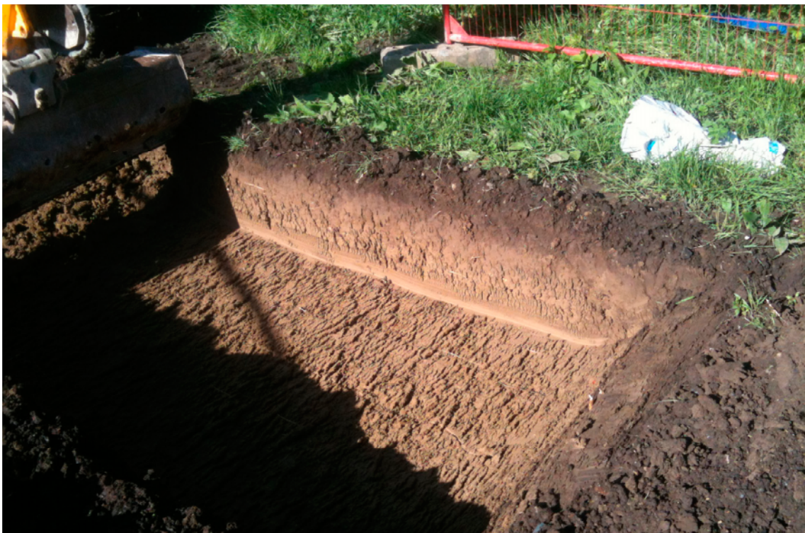
Plate 2. Drilling pit, looking southwest.
