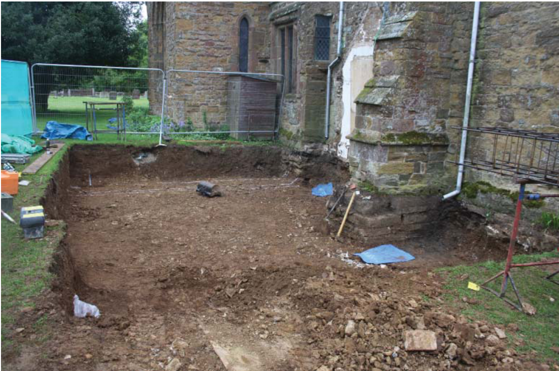
Plate 1. Site shot looking east.
