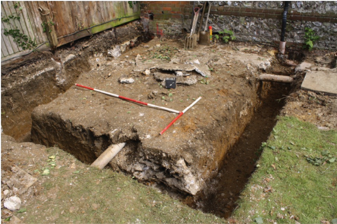
Plate 1. General view of footings, looking south-east, Scales: 2m and 1m.
