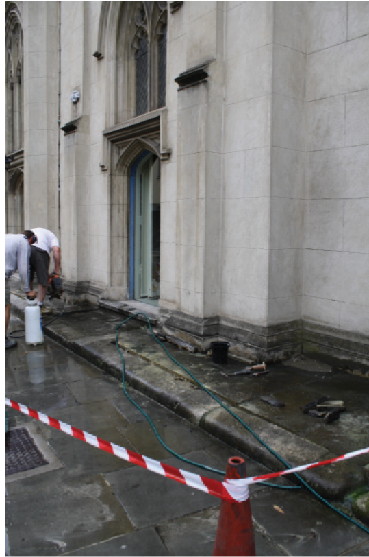
Plate 1. Area of investigation, looking north east.
