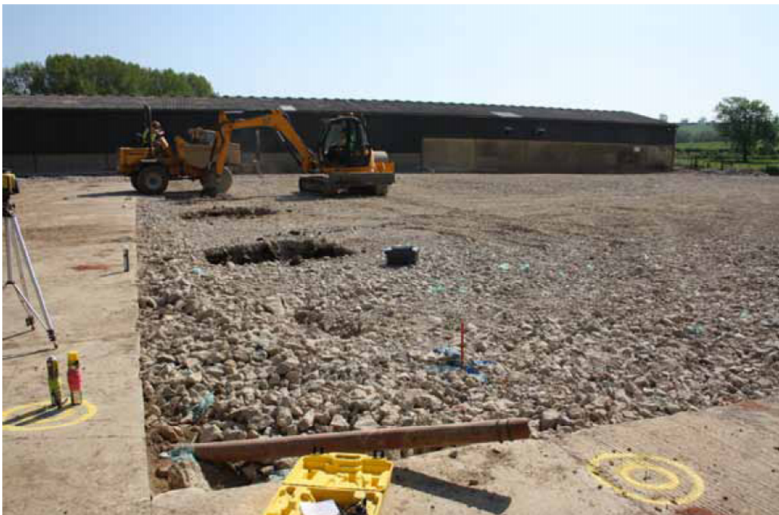
Plate 2. Excavation of pad for main barn in progress, looking east.
