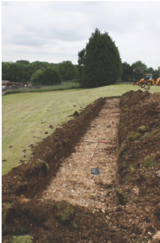
Plate 4. Trench 32, looking south east, Scales: horizontal 2m and 1m, vertical 0.3m.
